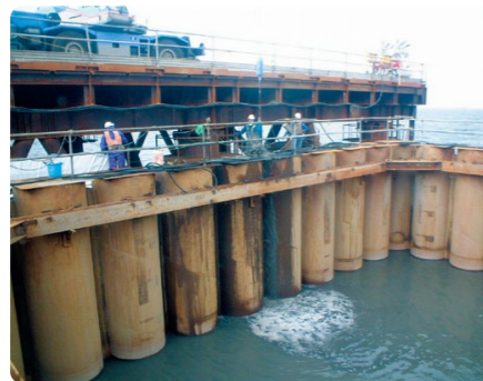
鋼管継手充填
